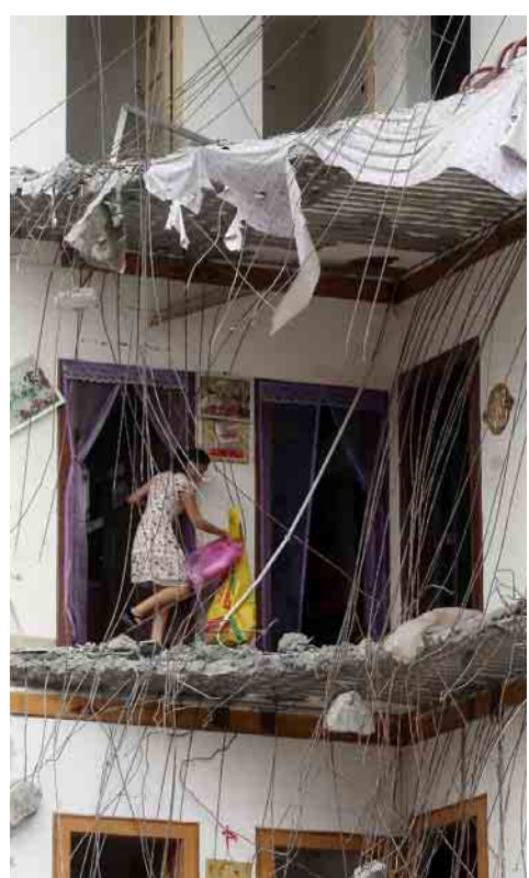
Thursday. A woman tries to make her way out of a partially collapsed building after an explosion caused by bombs hidden in parcels in Liucheng county, Guangxi (广西). Photo: Dickson Lee
